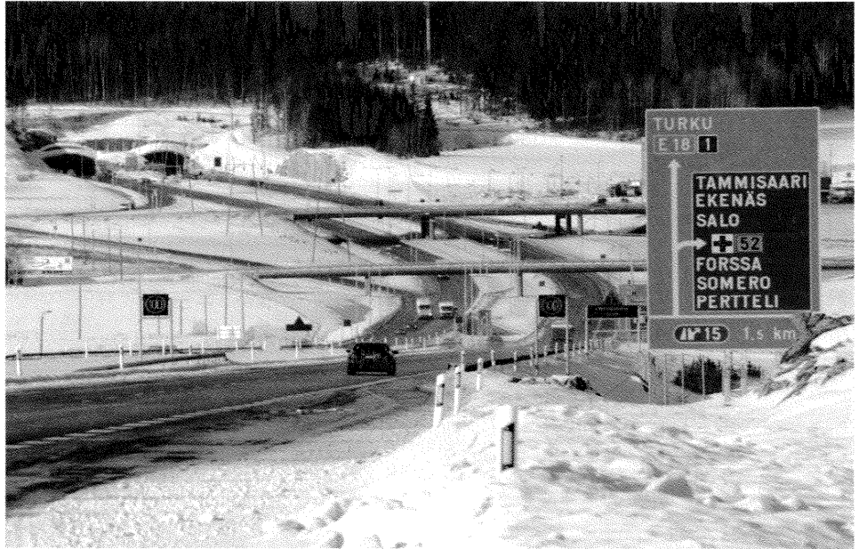
The E18 (Helsinki-Turku) motorway in Finland equipped with a weather-controlled speed limit system and variable slippery-condition warning sign, a good example of ICT deployment in traffic management and road safety. Developed by HIGHWAY consortium member Tieliikennelaitos (the Finnish Road Enterprise).
