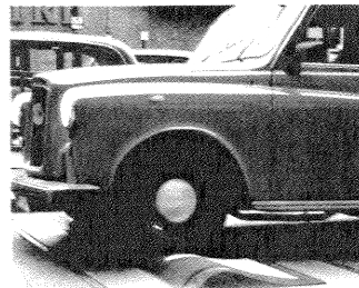
The Transcalm in operation: it does not affect 'safe speed' vehicles
